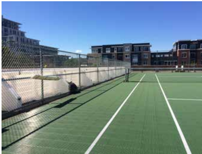
Tennis Courts on top of Reynolds Park Water Utility Building Photo by Jessi Mulhall
